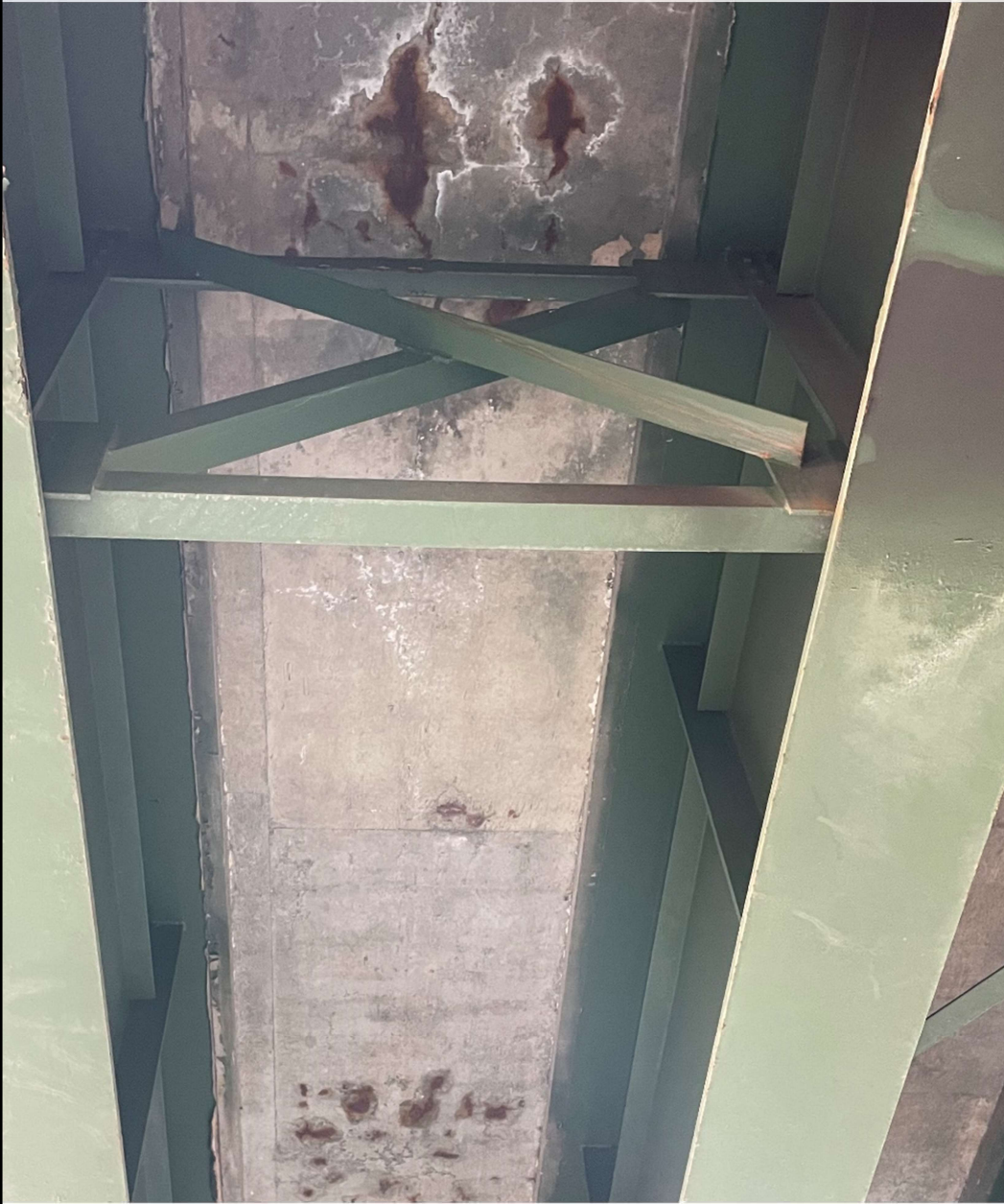
Spalling and Leaking Deck
